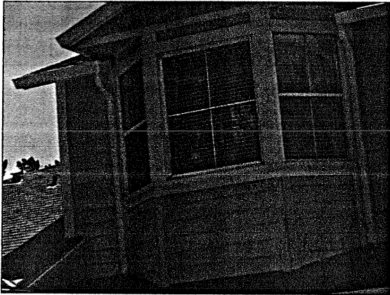
Exhibit 3: Hardboard Siding/Window Trim
