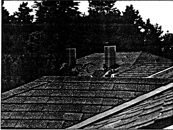
Exhibit 1: Comp Shingle Roofing
